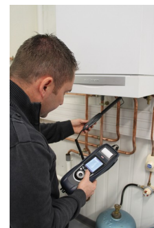
Ambient CO checking
